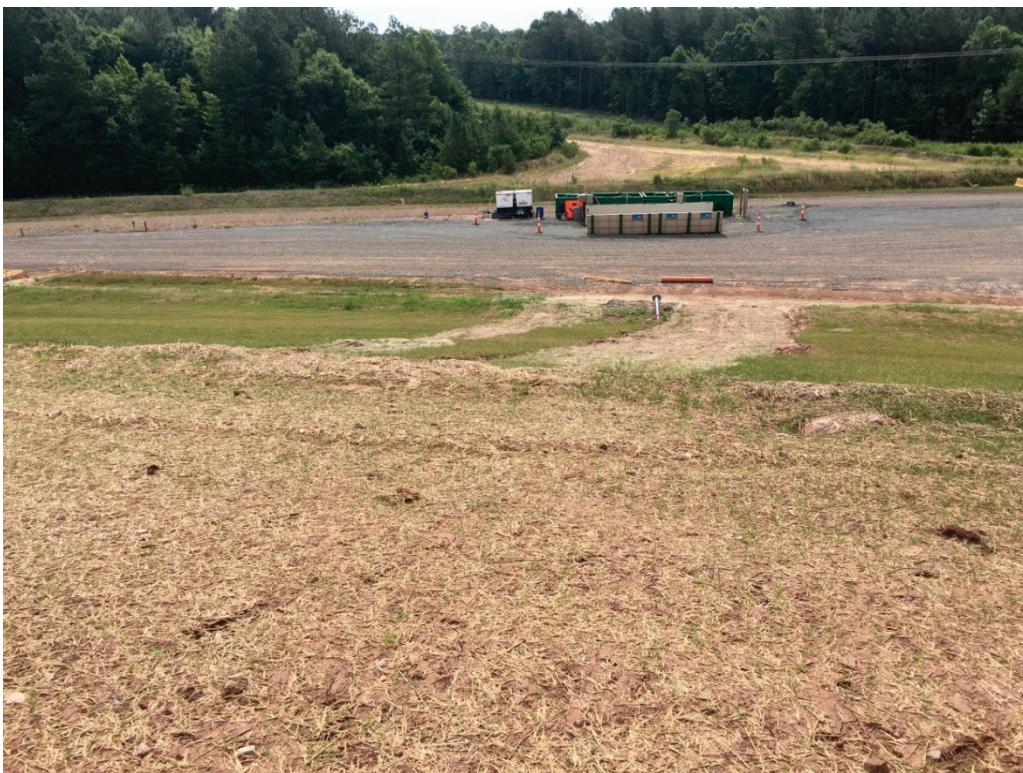
4. Erosion repairs on the eastern slope of Cell 1
