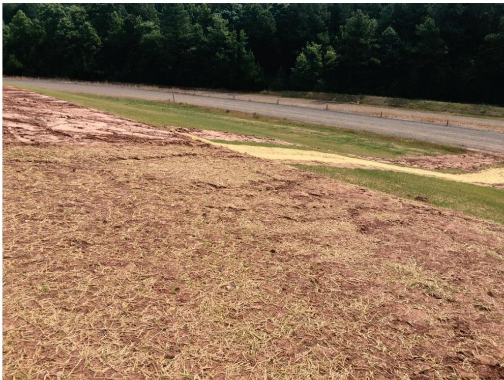
5. Erosion repairs on the eastern slope of Cell 1
