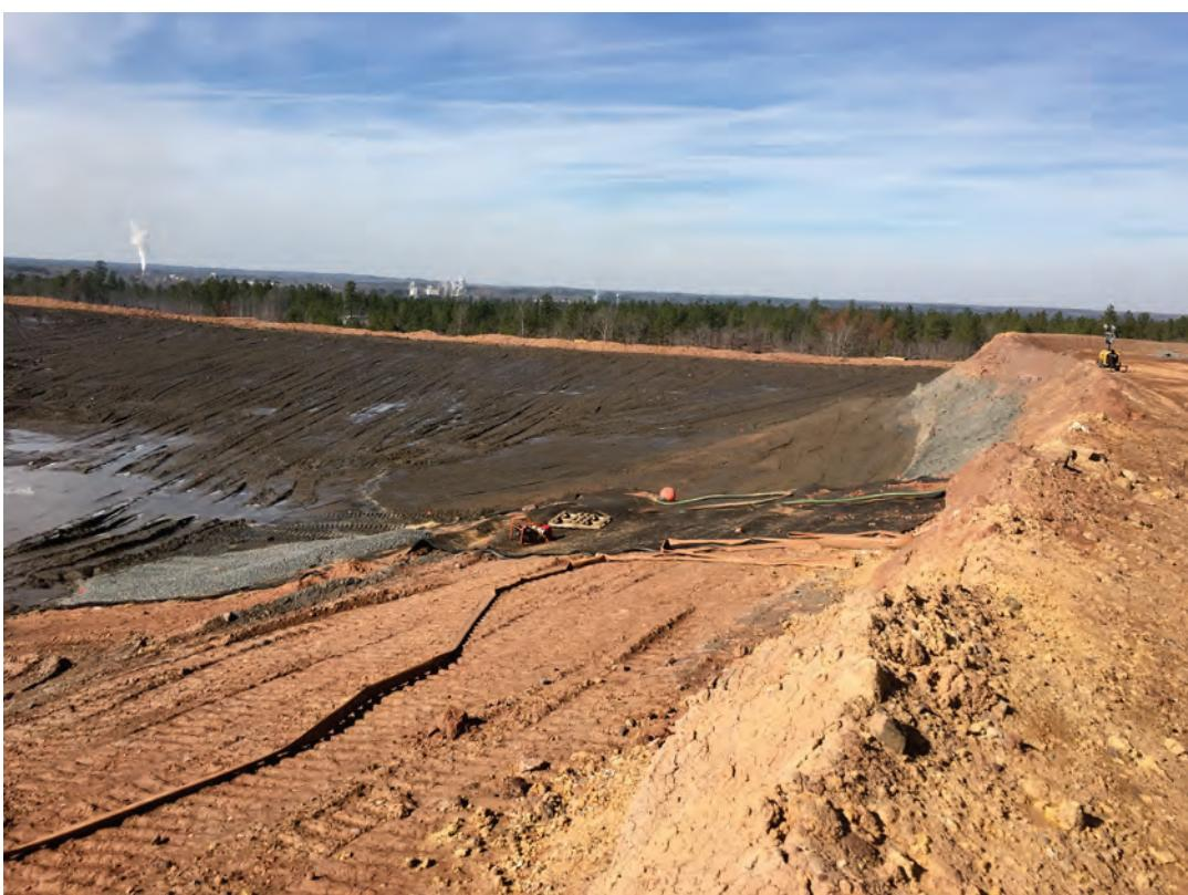
16. Divider berm to prevent run-on from capped areas into the ash
