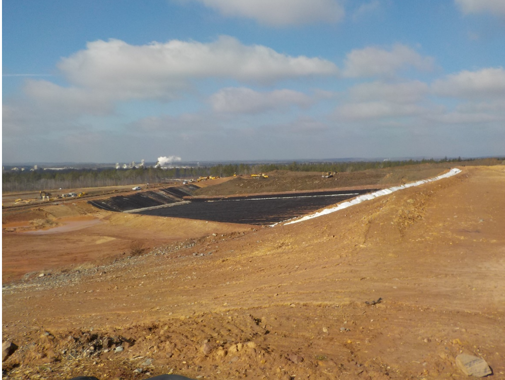
Photo 15 - Southern access road looking at 6C
