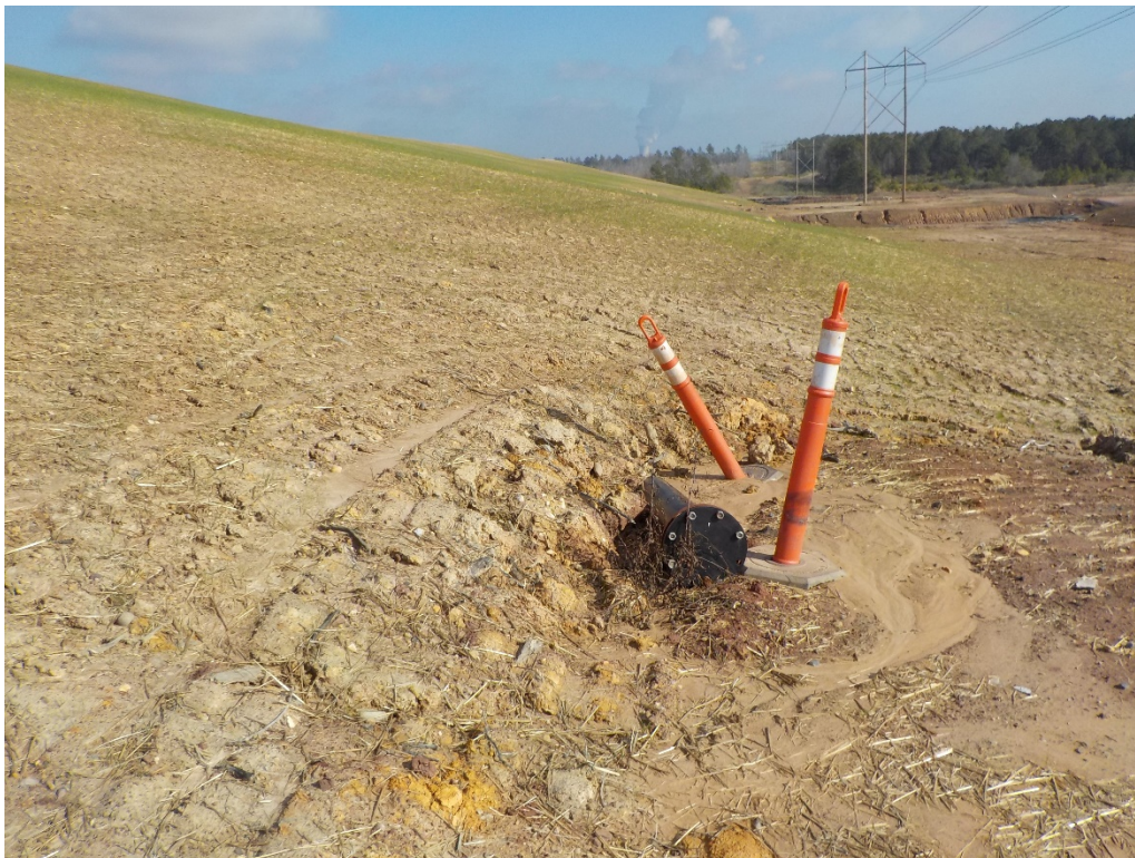
Photo 16 - Powerline row looking east
