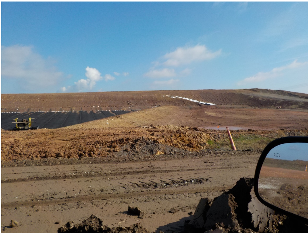
Photo 18 - 6C termination berm looking east
