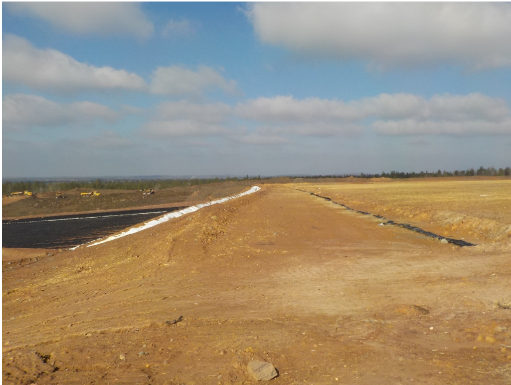
Photo 14 - Southern access road looking northwest at operations in 6B
