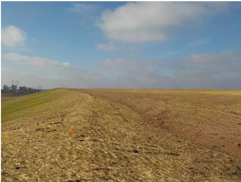
Photo 12 - Top deck diversion berm looking west
