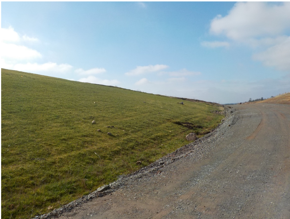
Photo 6 - Northwest corner looking west
