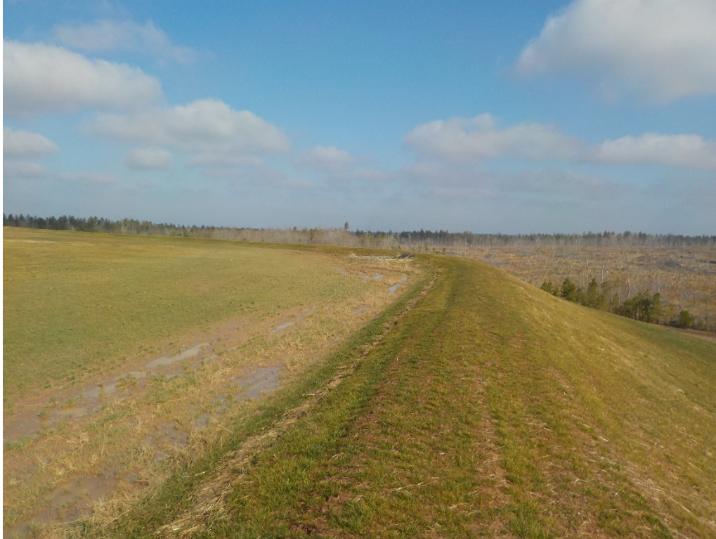
Photo 11 - Top deck diversion berm looking east at the slope drain
