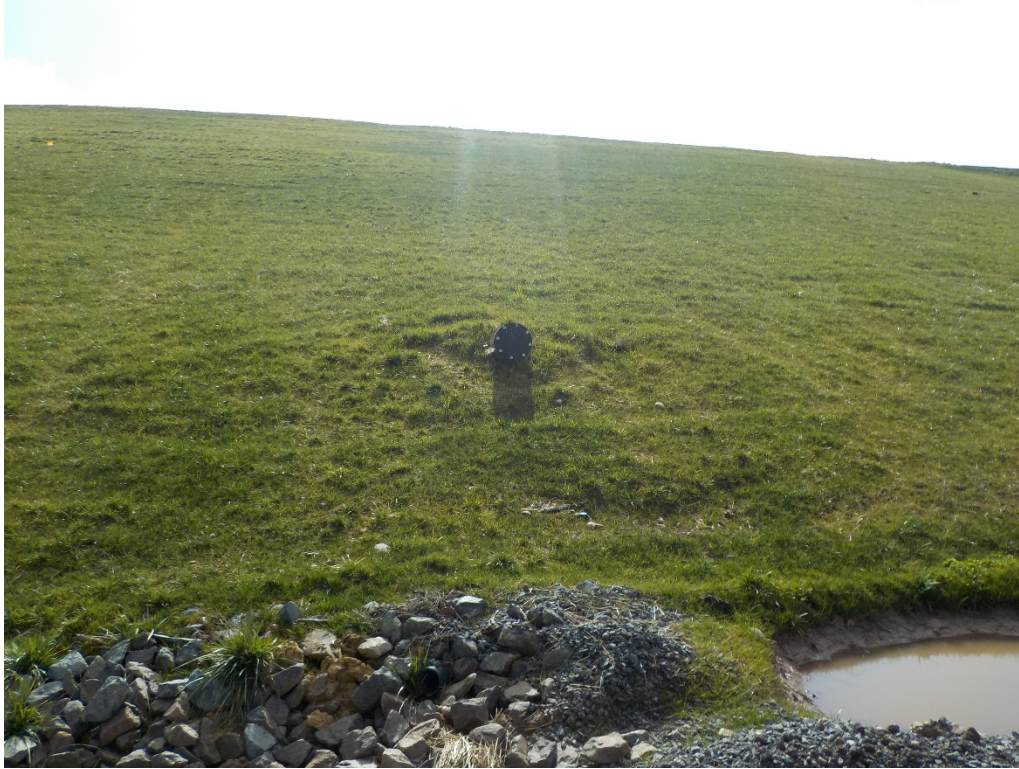
Photo 7 - Cleanout and toe drain
