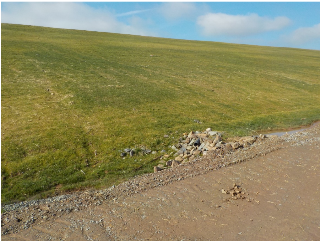
Photo 4 - East side toe drain looking northwest
