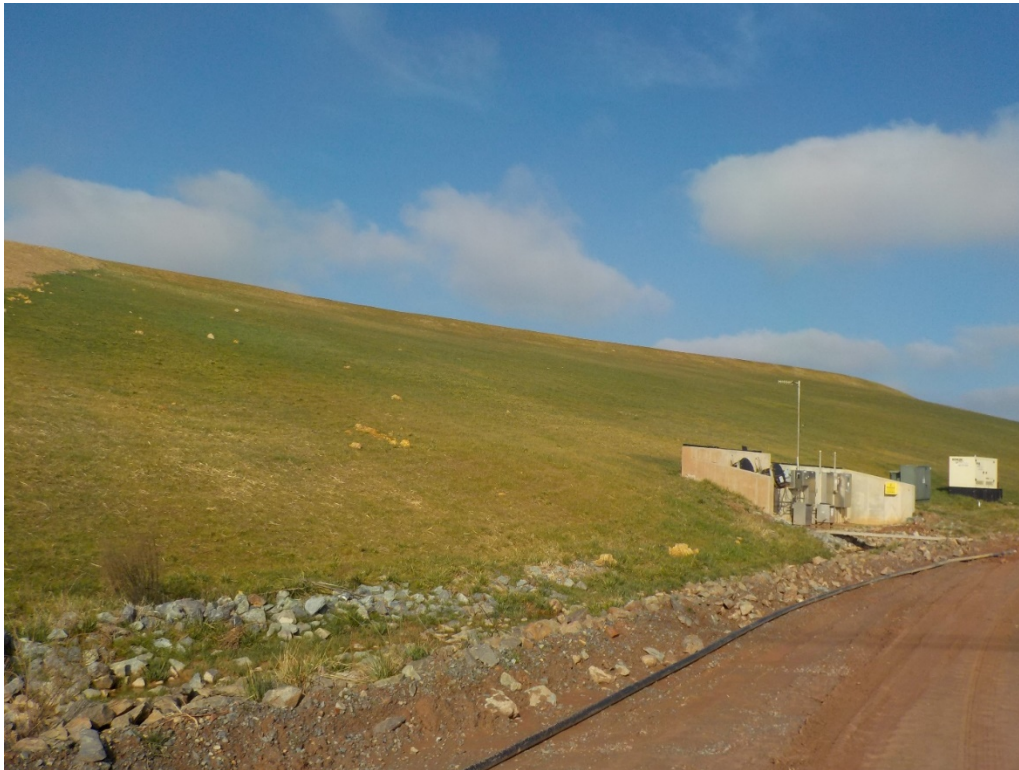
Photo 2 - Powerline row looking at Sump 1
