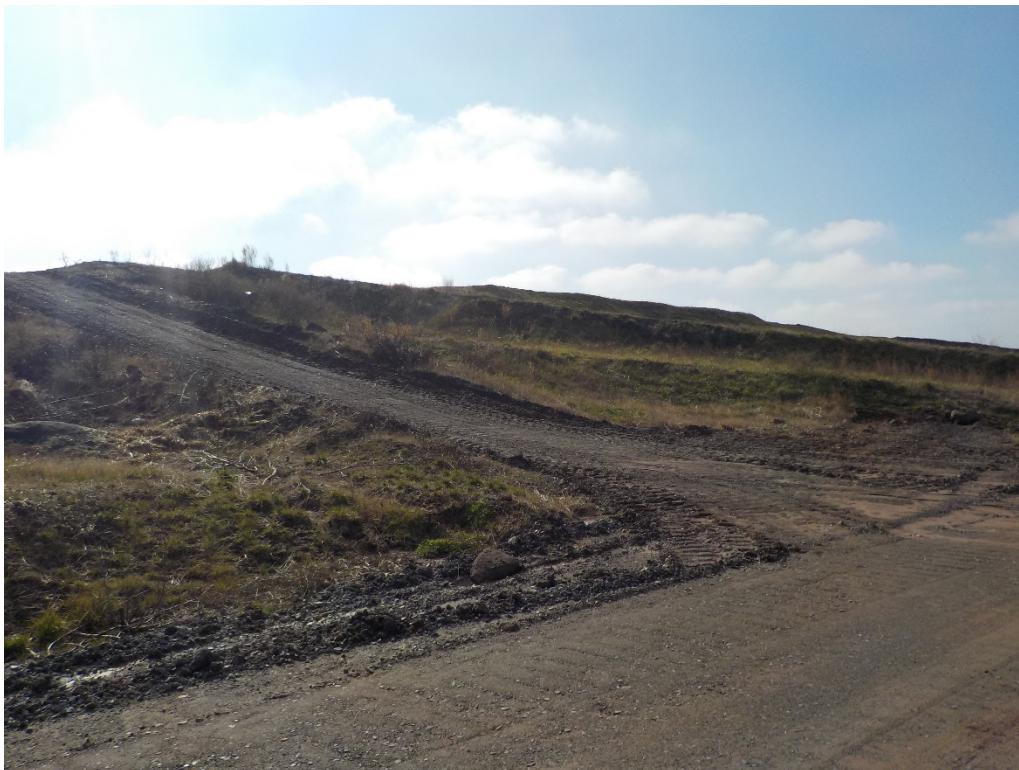
Photo 8 - Cell 1/2 access road
