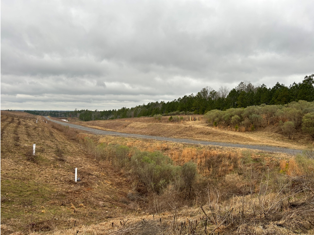
Photo 5 Top deck ramp looking west
