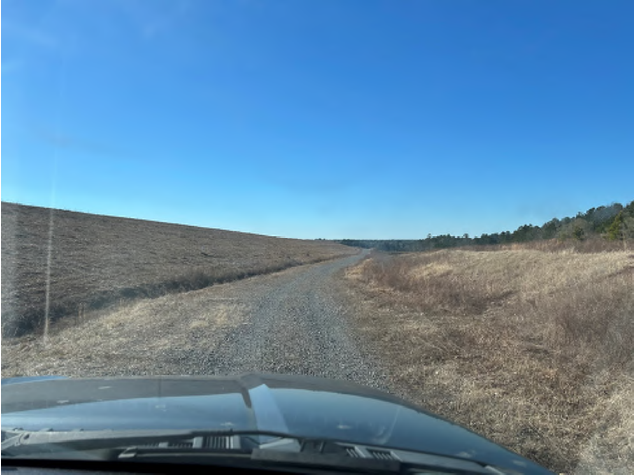
Photo 9 – Northeast Corner of the Perimeter Road Looking West
