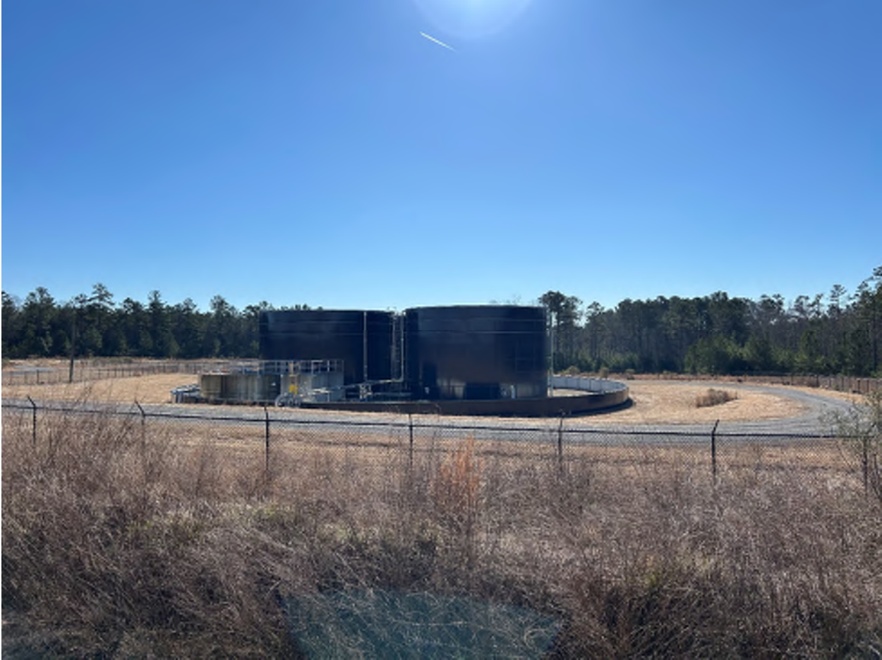
Photo 15 – Leachate Storage Tanks
