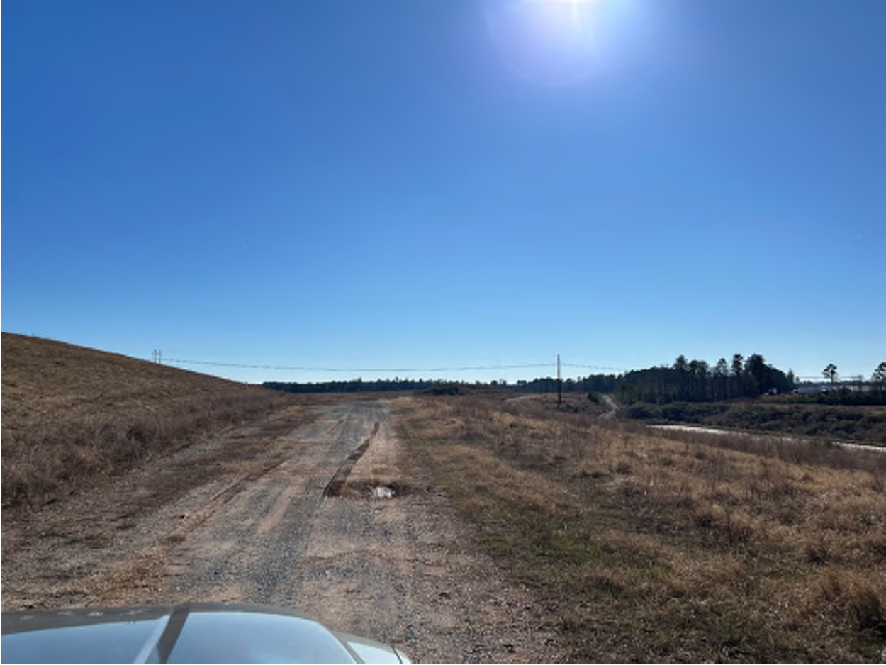
Photo 14 – East Perimeter Road Looking South
