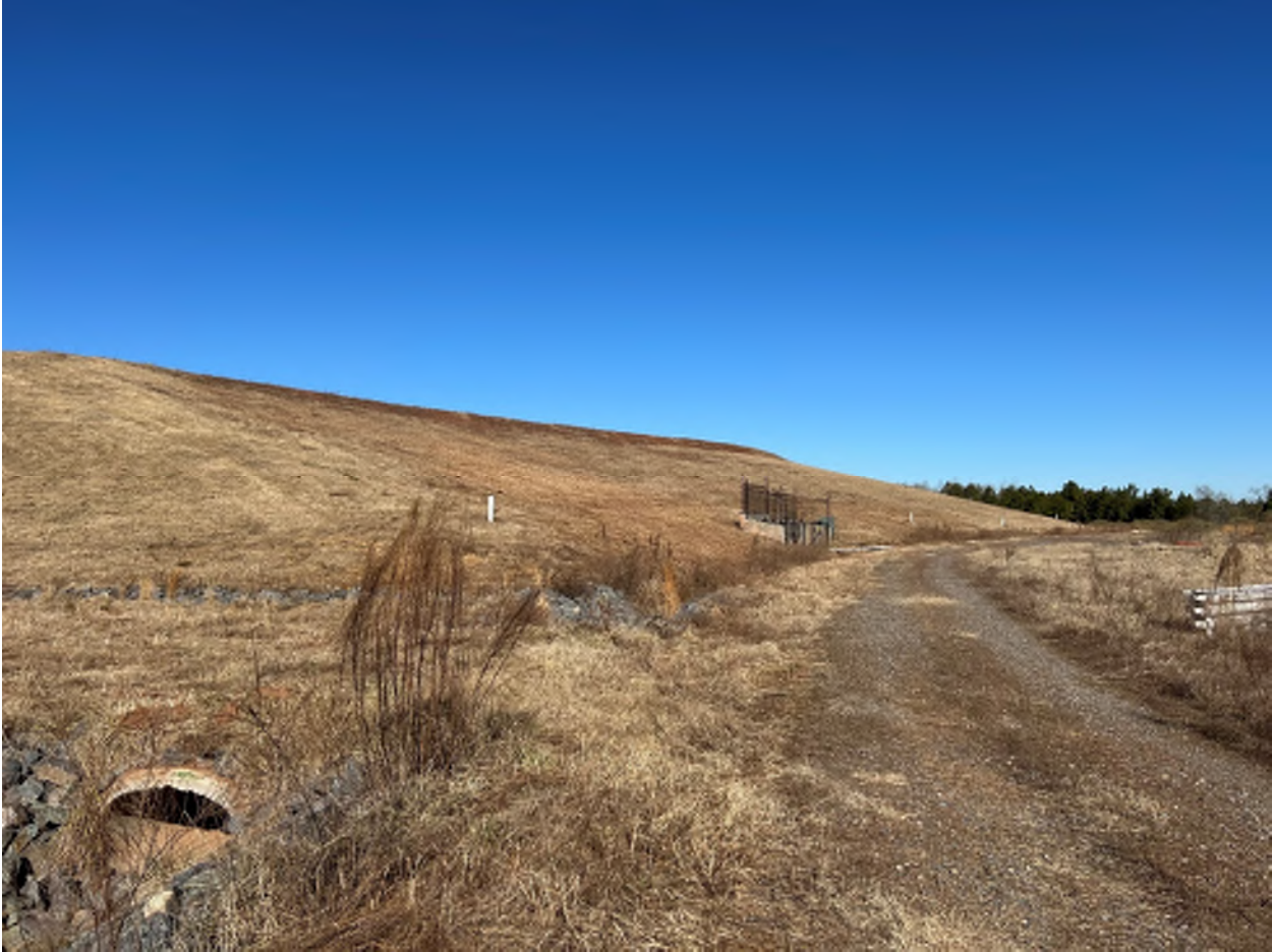
Photo 1 – Looking North at Sump 1
