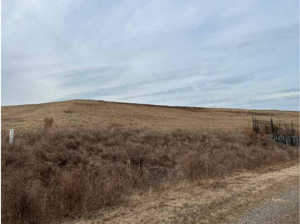
Photo 2 – Looking North at Sump 1
