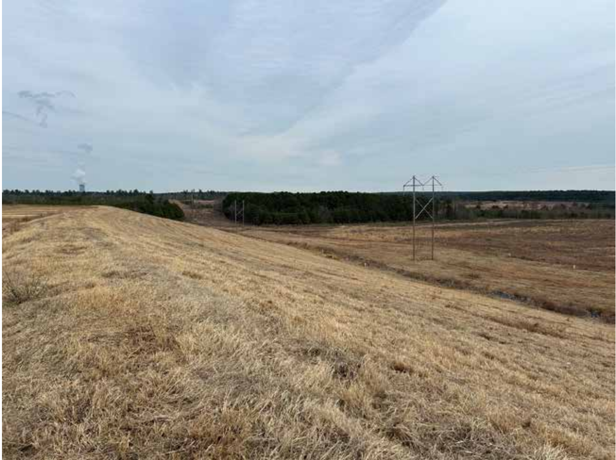
Photo 6 – Southern side slope of the CCR structural fill looking east toward sump 1
