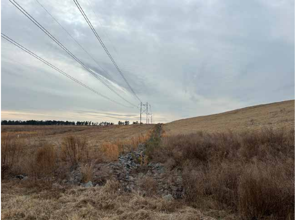
Photo 1 – Looking West at Sump 1
