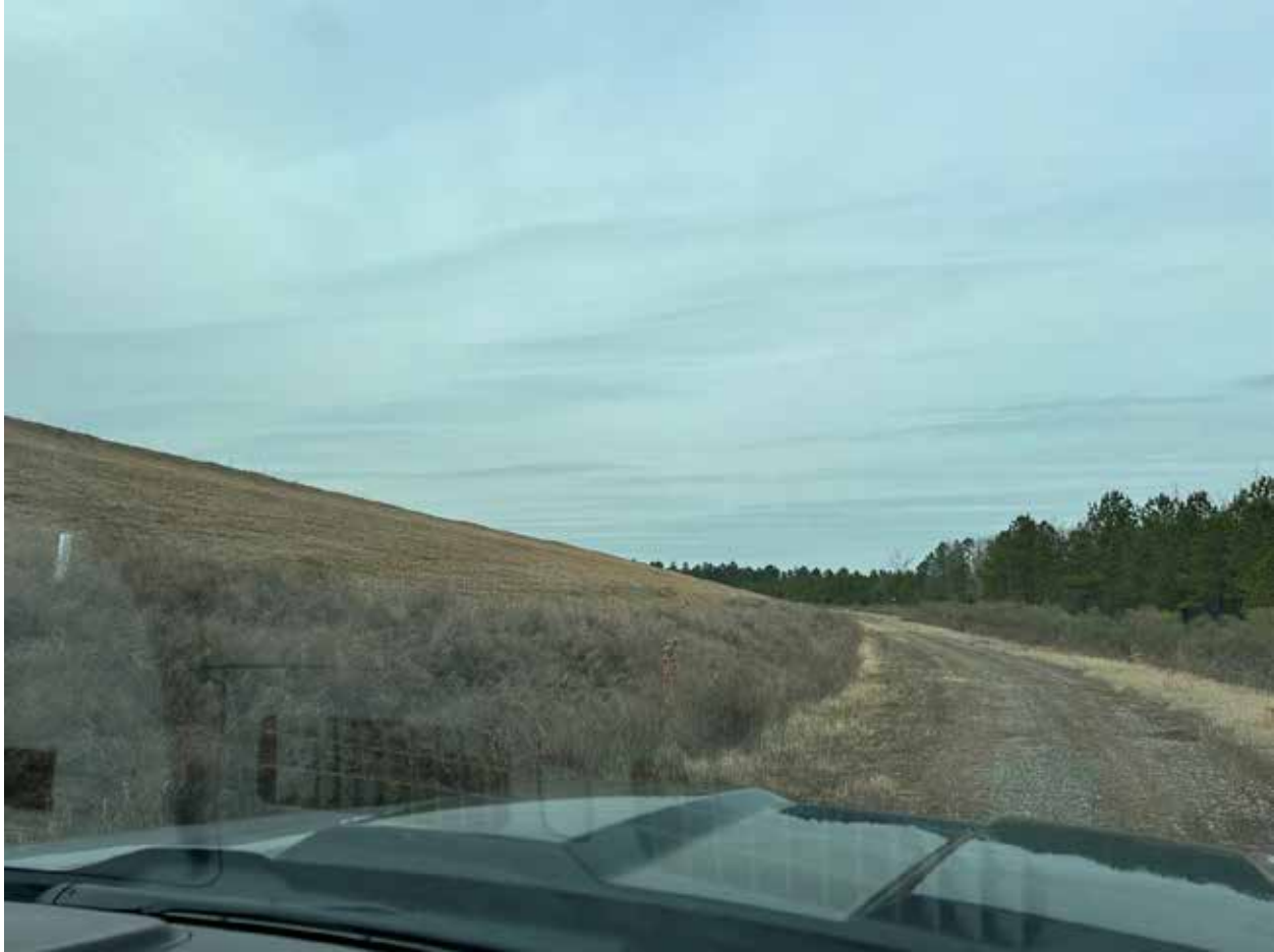
Photo 4 – Eastern side of the CCR structural fill looking north
