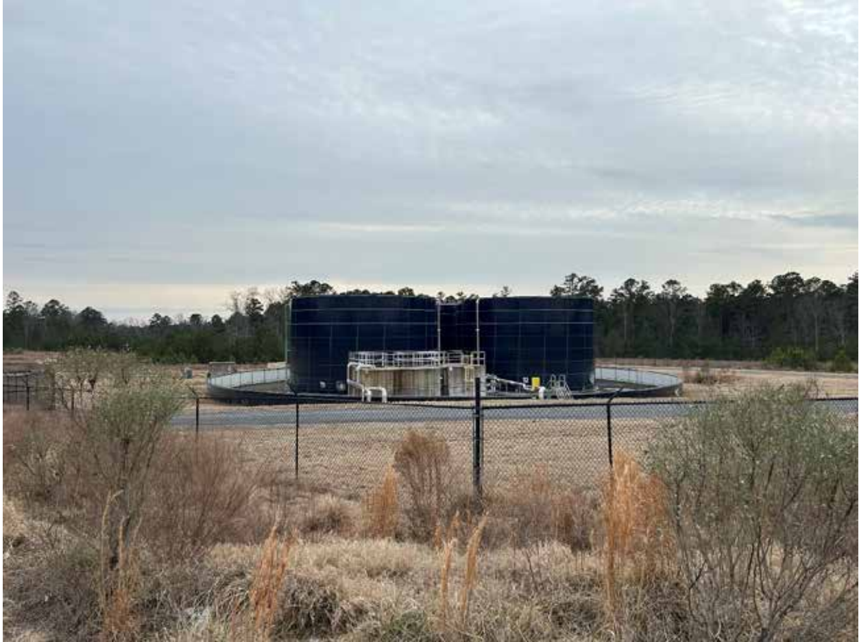
Photo 13 – Leachate storage tanks
